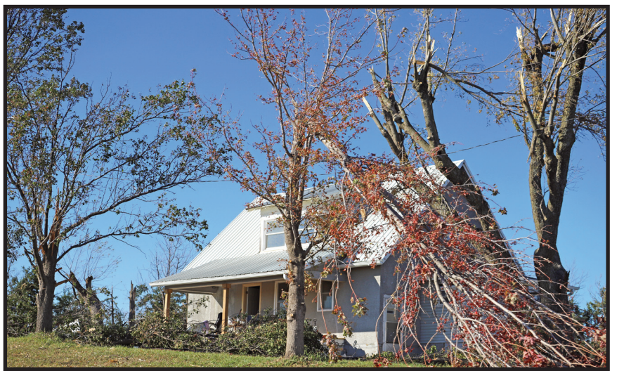
A home with damage near 656 Ave and 711 Rd.
