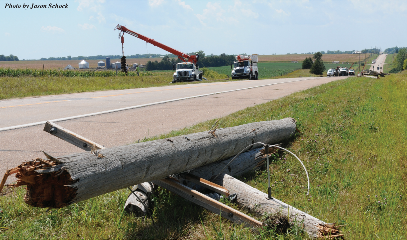
OPPD workers fix a series of broken powerlines along Highway 73 west of Verdon Lake July 26. The storm knocked down 15 69-kV transmission lines along Highway 73, between Humboldt and Verdon. Fourteen OPPD crews, along with crews from Falls City Utilities, worked all day and night Thursday, July 26, and restored power at 4:30 a.m. the following Friday. OPPD serves Falls City wholesale power from their 69-kV system, and when the transmission lines were down, OPPD had no way to provide service to their substations, resulting in outages on five OPPD Circuits for a total of 1,325 retail customers and two OPPD wholesale customers - Magellan Gas and Falls City Utilities.
